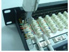
Press foil or braid shield to contact ground, and keep the cable straight;
